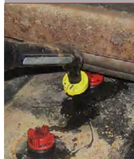
Manual watering guns cannot reach back row of cells when installed
